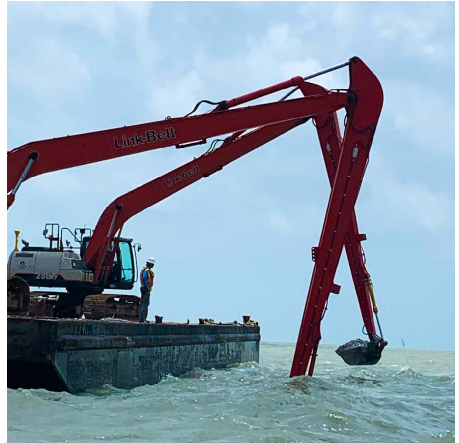
Oyster reef construction (Texas Parks and Wildlife Department).
