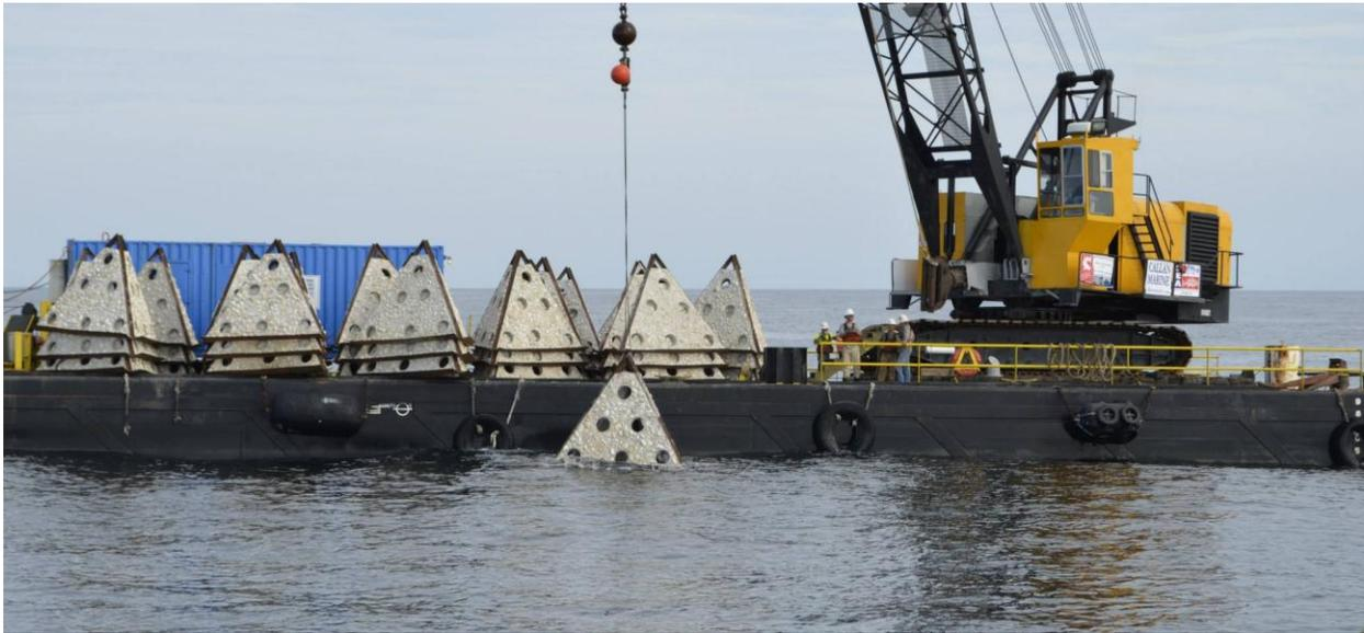
**Figure 8-6. Photograph of previous artificial reef material deployment completed in Texas.**
